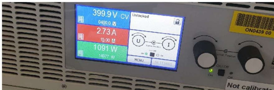
Figure 23. DC Power Supply Reading @ 1 kW.
